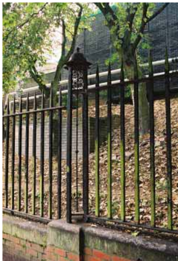
Listed railings, Lovers Lane
